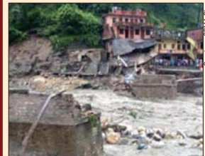
Gangotri bridge in Uttarkashi damaged due to flash flood in August.
